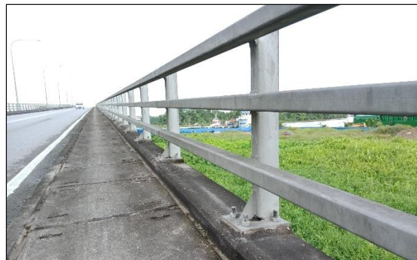
Figure 11. Standard Curb with Steel Railing.
