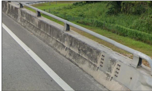
Figure 12. New Jersey Parapet with Steel Railing.
